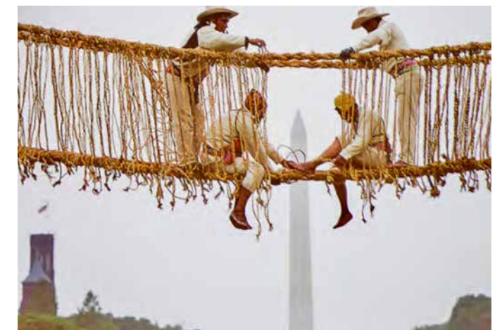
Utilizing traditional Inka techniques, Andean specialists construct a fiber suspension bridge on the National Mall, Washington, DC.
